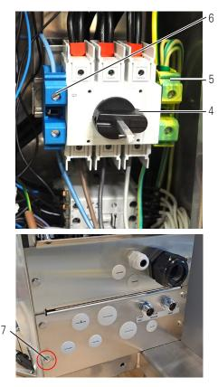
Detach the lead-through plate (2) from the pillar. Slip the supply cable (1) through the cable bushing (3) of the lead-through plate. Connect the phase wires of the cable to the mains switch (4) and PE and N cables (5, 6) to the terminal blocks.
